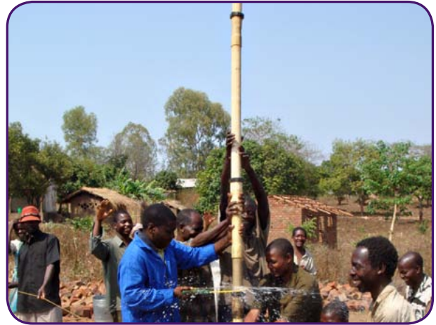
Figure 8: Working with a community-based organization to rehabilitate a hand pump for a village well in Malawi
